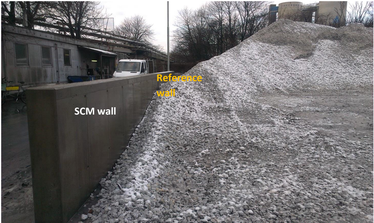
Figure 5. Visual aspect of walls on 21-Jan-15
