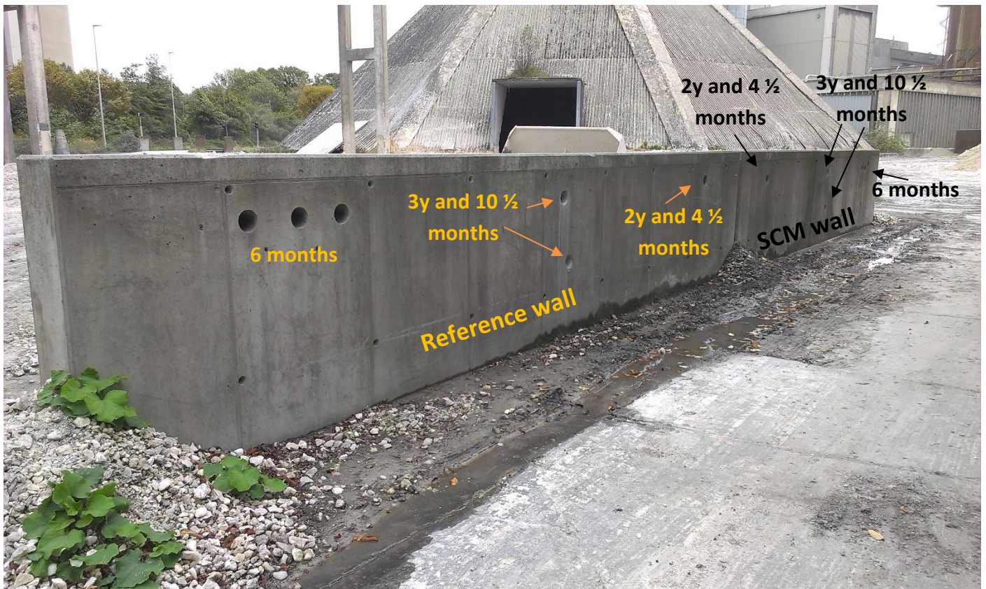
Figure 6. Location of drilled concrete cores and visual aspect of walls on 19-9-18
