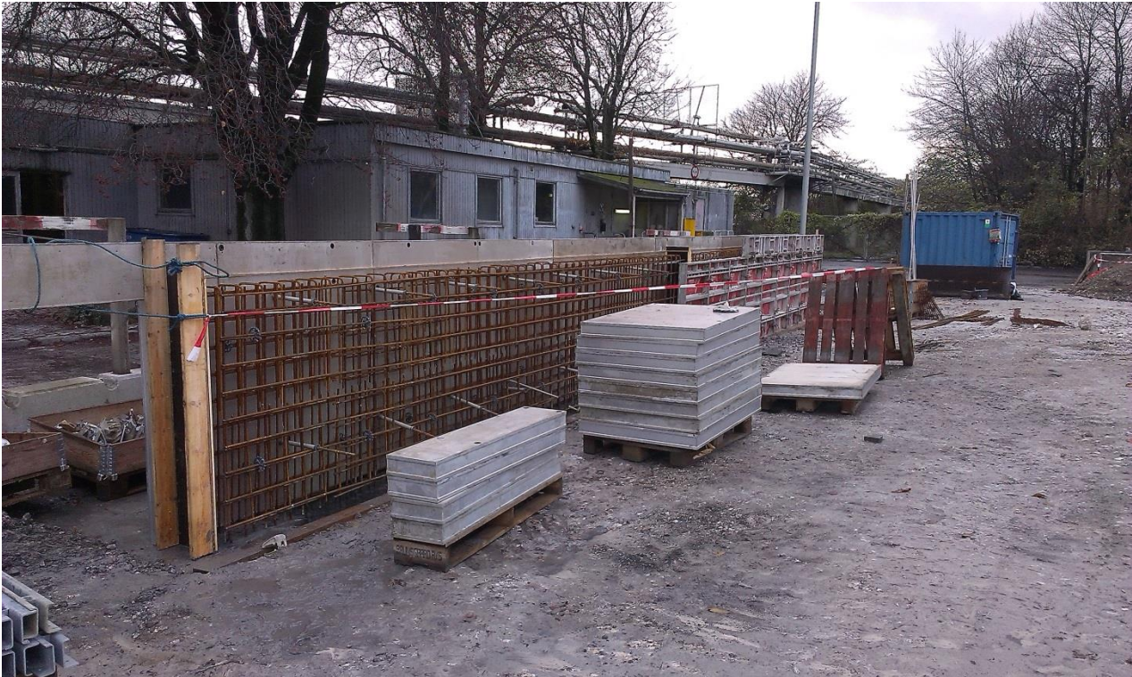
Figure 3. Reinforcement and formworks
