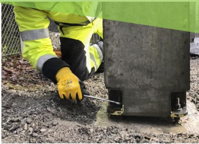
FIGURE 3 BOLTED PRECAST COLUMN CONNECTION WITH HIGHLIGHTED RECESS BOXES
